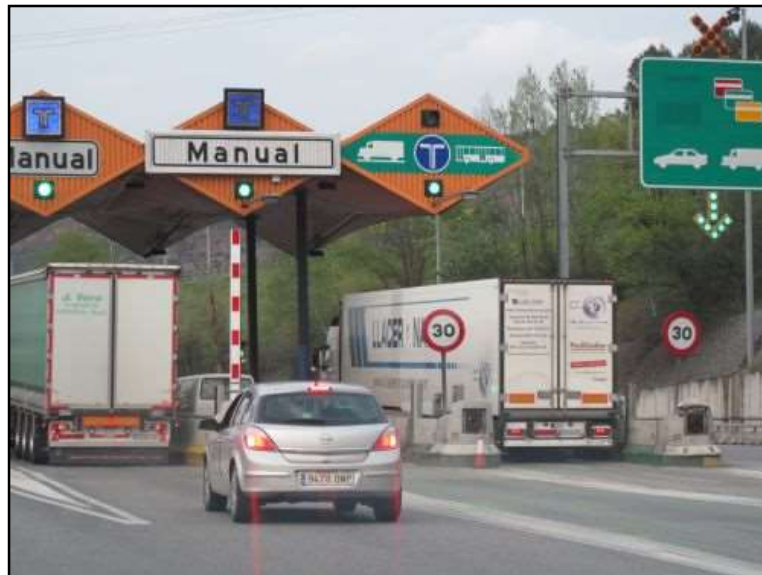
Example of a VIA-T station
